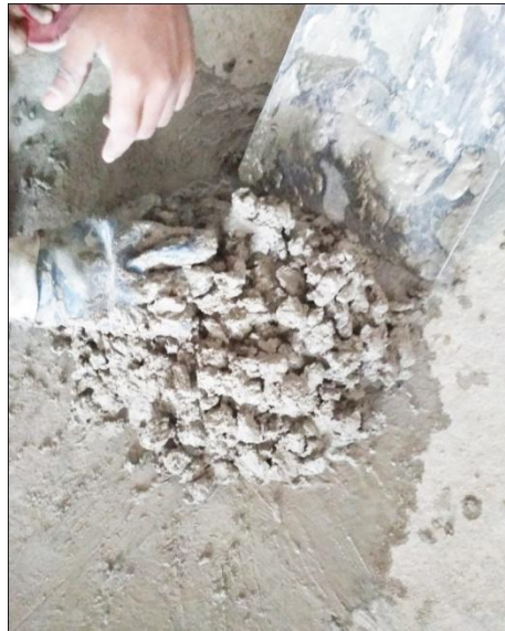
Figure 5.3.2.1(a): Mixing of concrete
